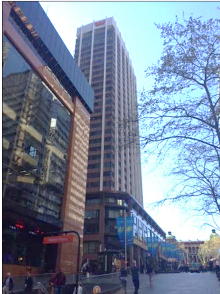
Figure 2: View of the existing commercial building as viewed from Martin Place looking east
