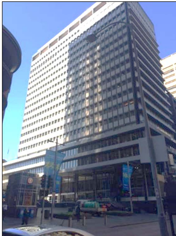
Figure 11: View of the Reserve Bank building from Martin Place
