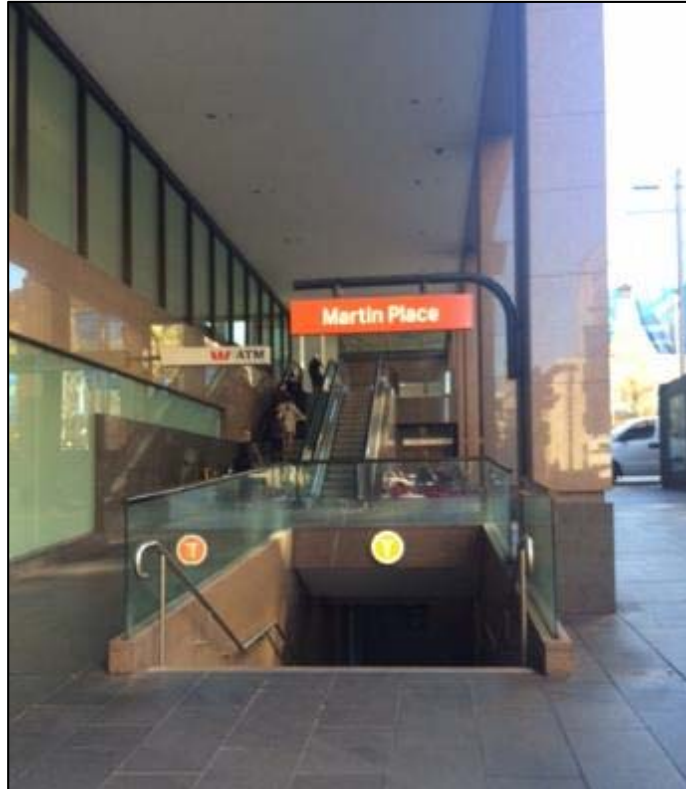
Figure 7: View of the existing station entry stair to be replaced as part of this application
